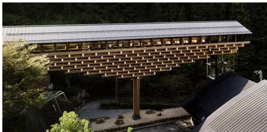
図 15. Kuma Kengo. Yusuhara Wooden Bridge Museum, 2010
